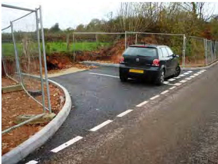
Figure 3.7 – Newly Constructed Access to Area B
